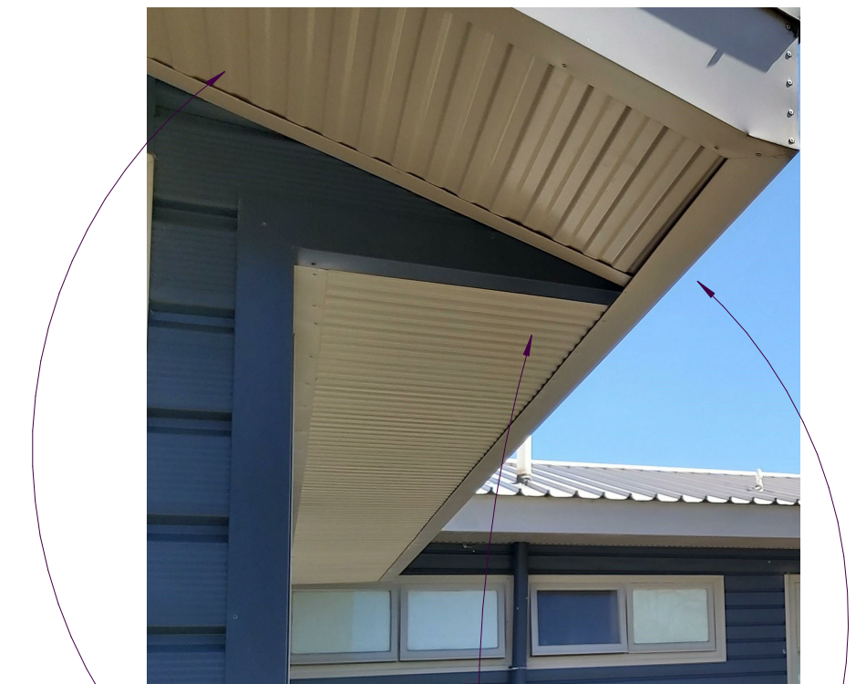
Photo C Proposed Eave Boxing In Colorbond
